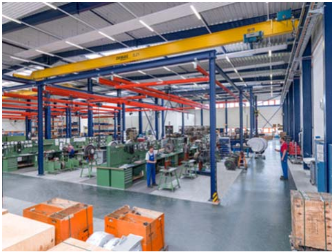
Figure 3: Free standing supporting structures
